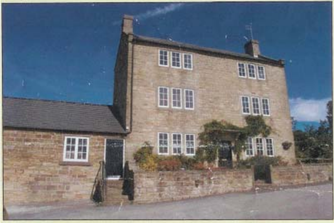
This is Amberley Farmhouse, a Grade II listed building in Pentrich.
